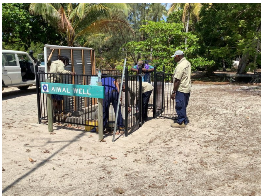
Figure 16: Warraber’s Aiwal Well is a concrete lined square well with a total depth of 2.89 m bgl.
