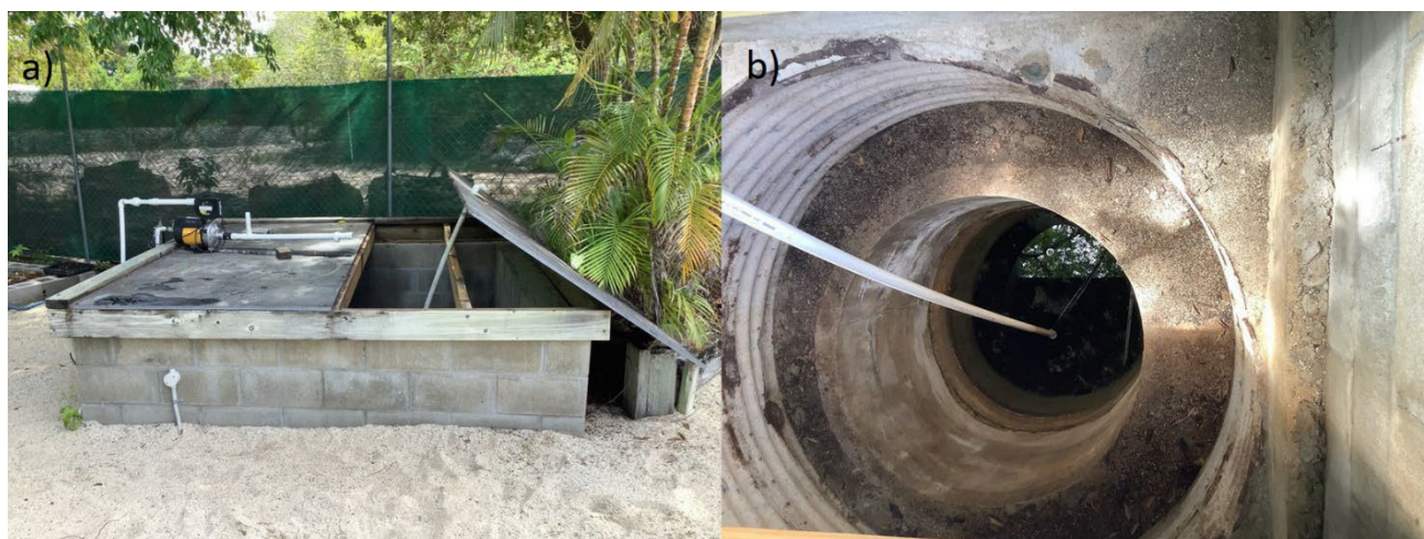
Figure 23: Mother's Well is a concrete lined circular well located on Masig Island at the Mothers Well Nursery. The well has a total depth of 6.0 m bgl.
