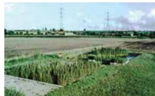
Constructed wetland on a farm for agricultural effluent treatment
